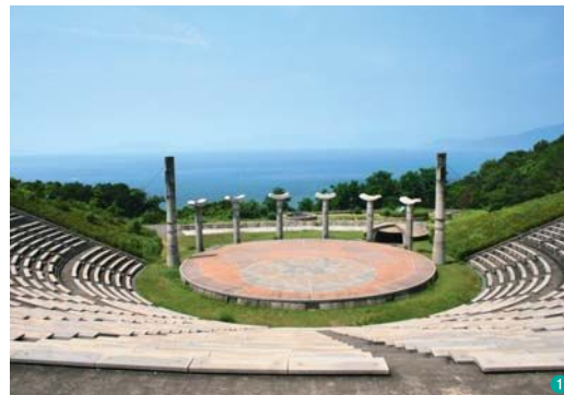
1 Sanuki City Outdoor Music Space Theatron 2 Sanuki Winery 3 Sanuki City Produce Center
